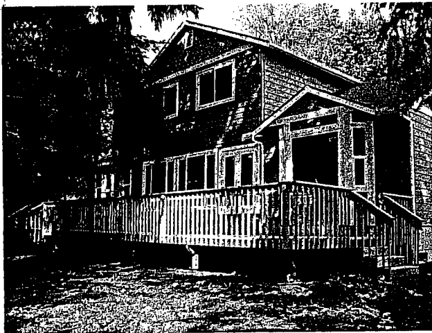
REAR VIEW OF THE HOUSE
