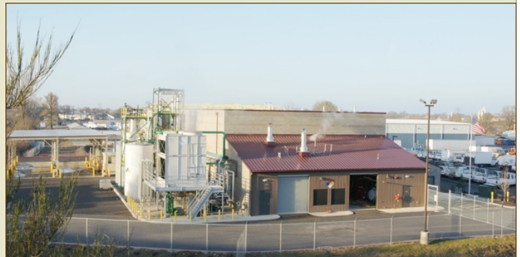
Sequential Pacific Biodiesel plant on Turner Road in SE Salem
