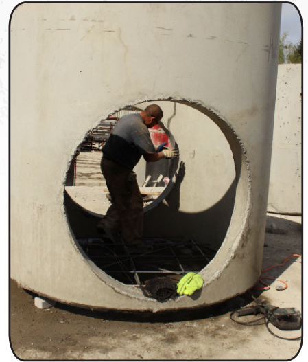
The Keizer company reuses its hole formers thousands of times and eliminates tons of excess concrete waste.
