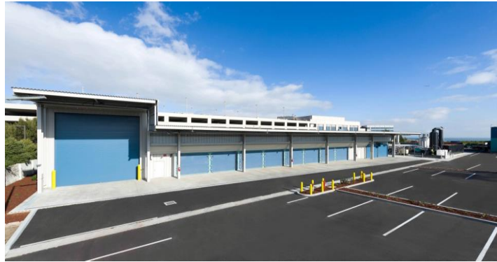
(Pictured above; Blueline AD – CNG Fueling Station)
