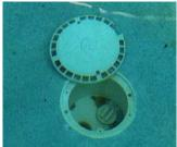
Floor drains that are cracked, chipped or no longer screwed in must be corrected immediately before the pool can open
