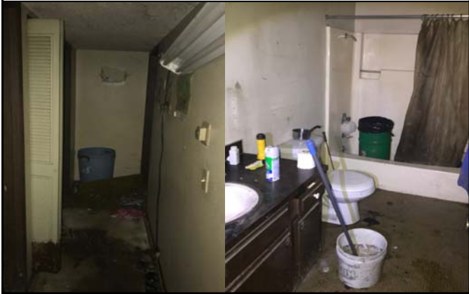
Hallway and Bathroom: R88709
