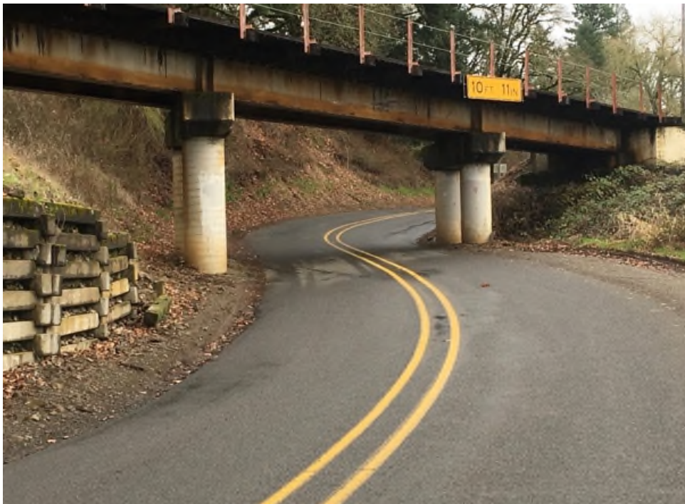
Figure 10. Railroad Overcrossing Structure on Riverside Drive – Southbound View (See 20 in Figure 8)
