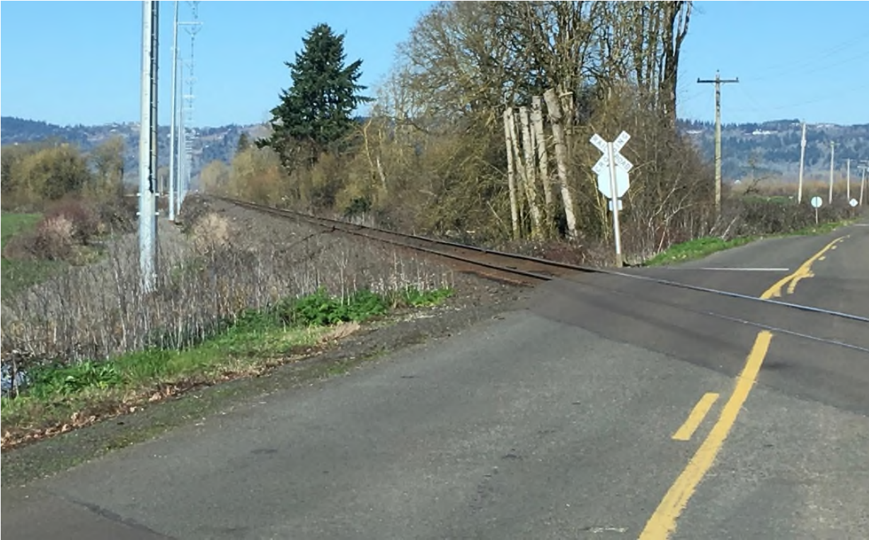
Figure 28. NB on Marlatt Road Crossing 3E-87.5 Looking left (See 17 in Figure 8)
