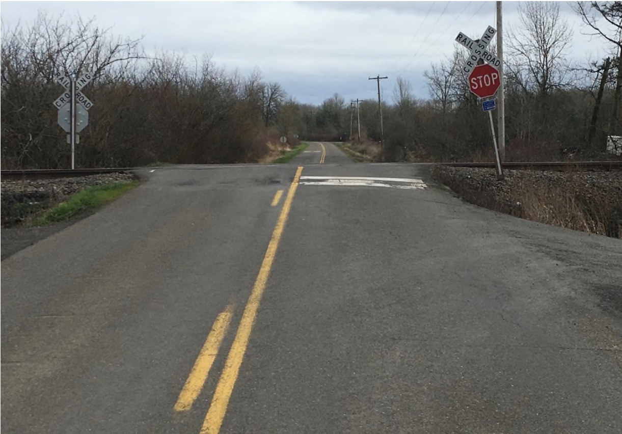
Figure 23. EB on Wintel Road Approaching Crossing 3E-86.8 (See 18 in Figure 8)
