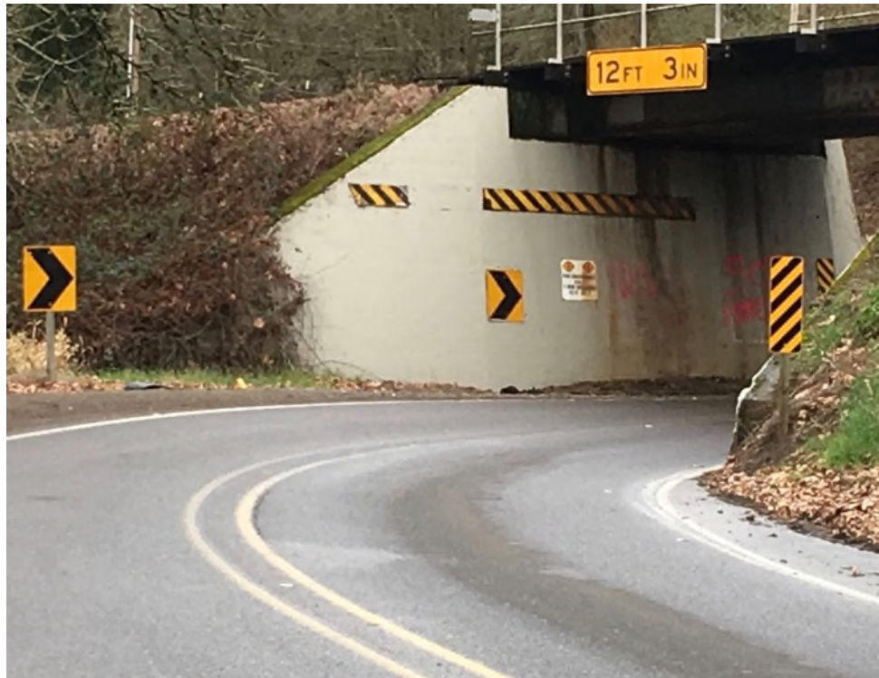
Figure 13. Railroad Overcrossing Structure on River Rd - Northeastbound View (See 21 in Figure 8)
