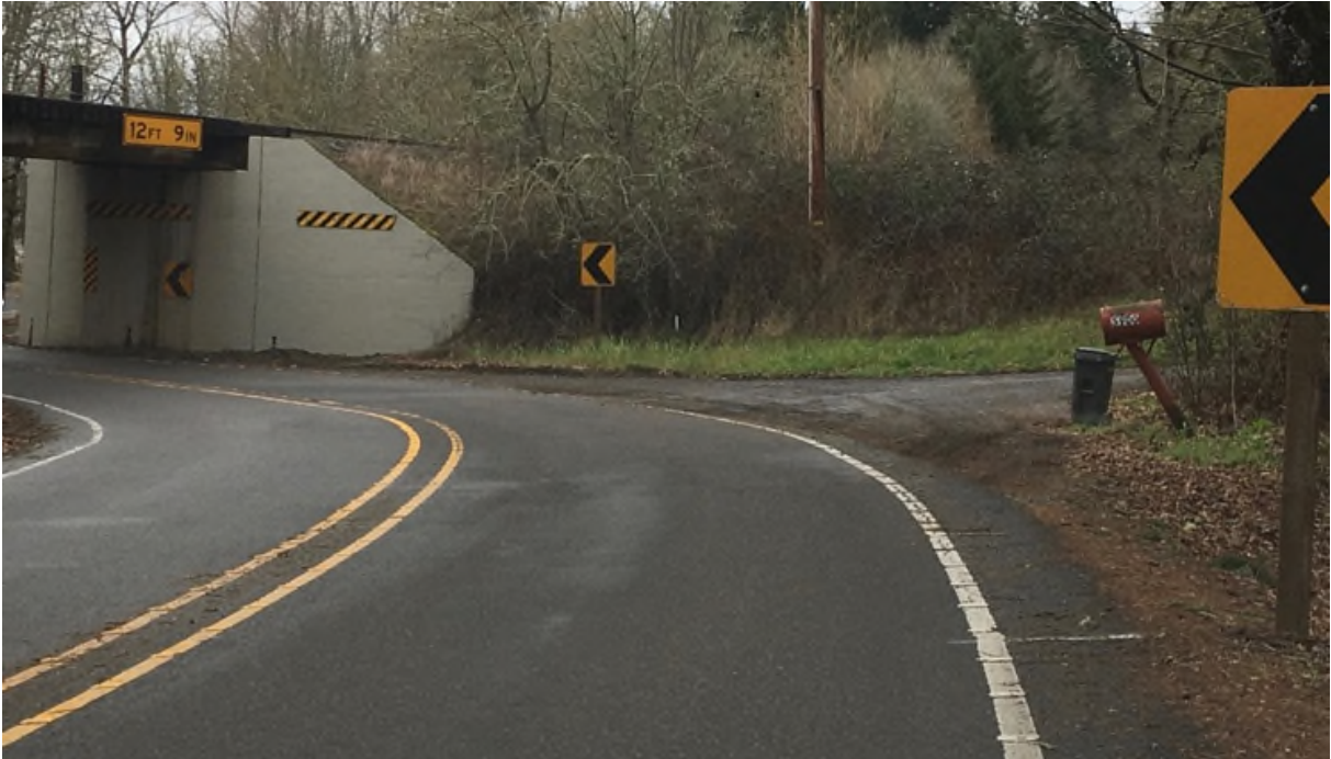
Figure 15. Railroad Overcrossing Structure on River Rd - Northeastbound View (See 22 on Figure 8)
