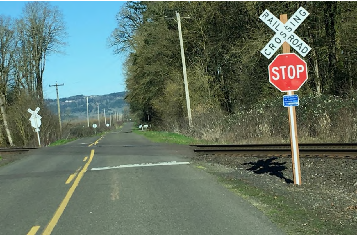
Figure 27. NB on Marlatt Road Approaching Crossing 3E-87.5 (See 17 in Figure 8)
