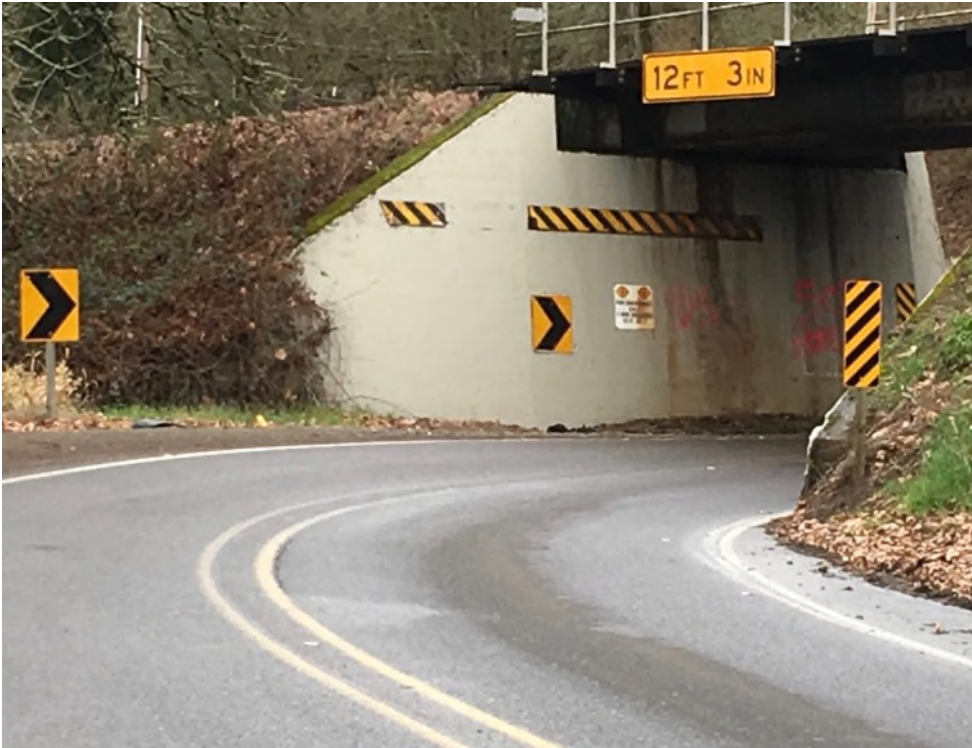
Figure 15. Railroad Overcrossing Structure on River Rd - Northeastbound View (See 21 in Figure 10)
