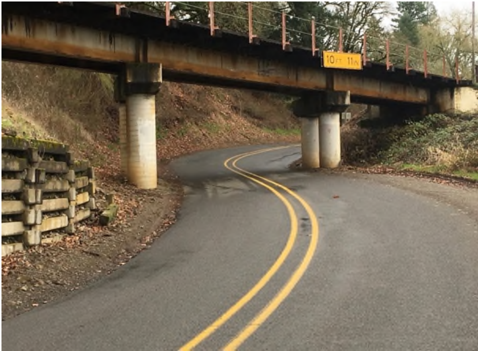
Figure 12. Railroad Overcrossing Structure on Riverside Drive – Southbound View (See 20 in Figure 10)
