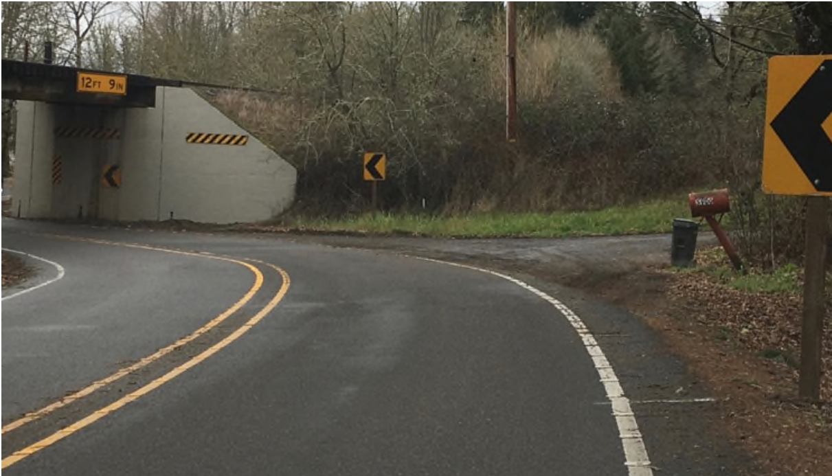
Figure 17. Railroad Overcrossing Structure on River Rd - Northeastbound View (See 22 on Figure 10)
