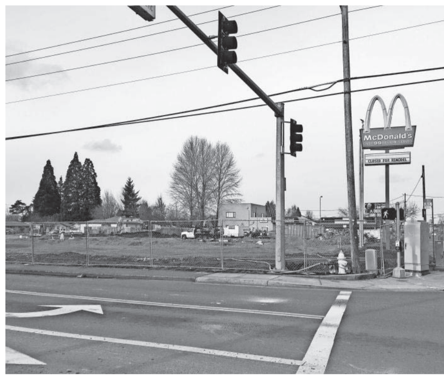
Construction work at the site of the McDonald's restaurant at 1011 Lancaster Drive NE in Salem on Jan. 31. LEE CLARKSON/STATESMAN JOURNAL
