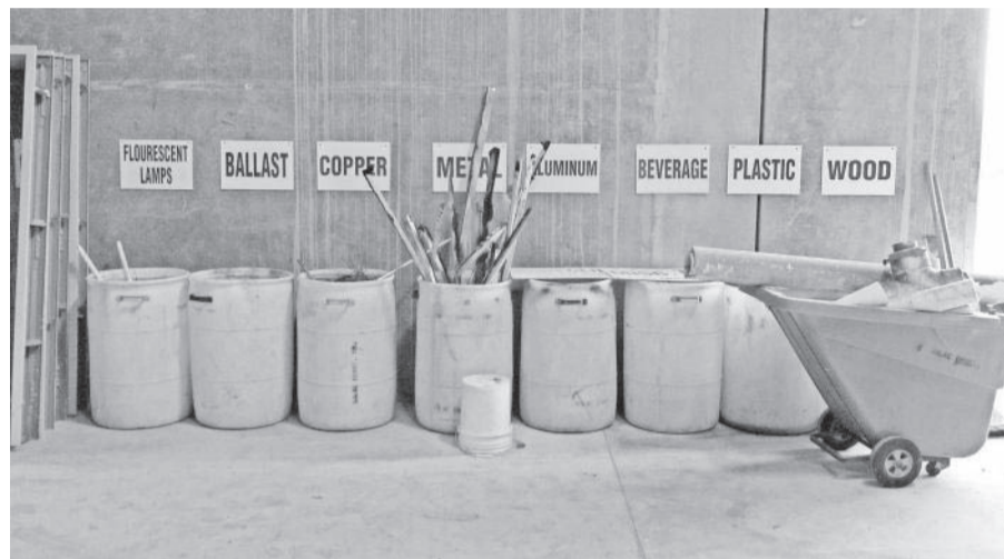
Separating out construction materials at work sites is part of Dalke Construction's waste reduction efforts. SPECIAL TO THE STATESMAN JOURNAL
