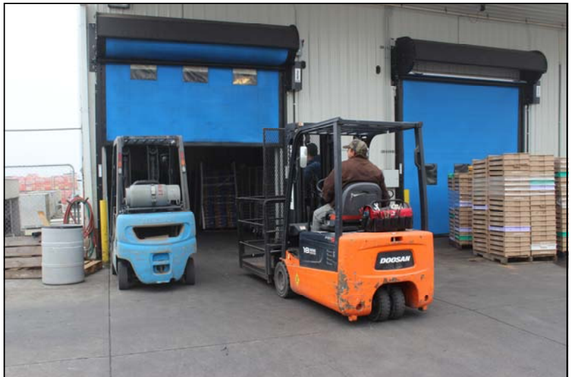
Automatic high-speed roll-up doors allow for faster forklift loading
