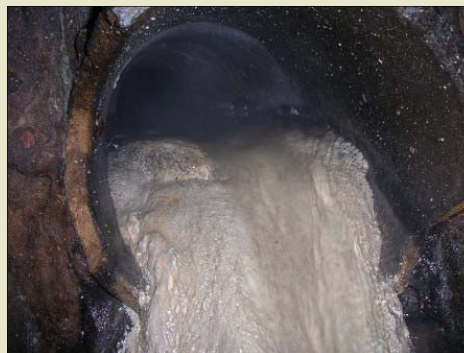
An example of a cascading fatberg.
