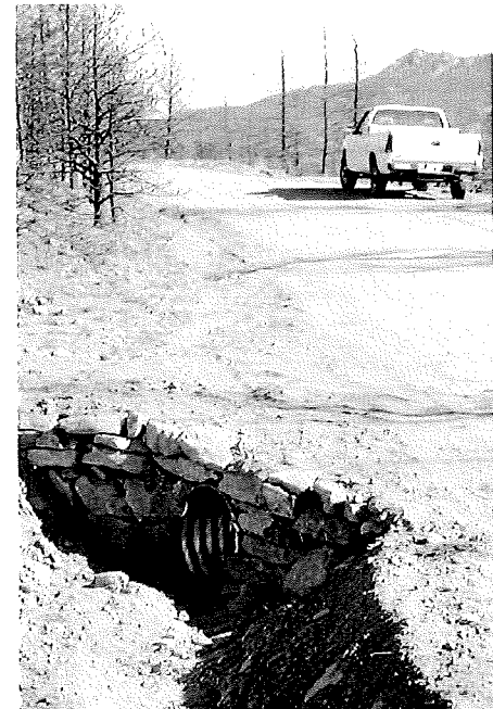
To be effective, culverts must be installed properly and at proper locations.
